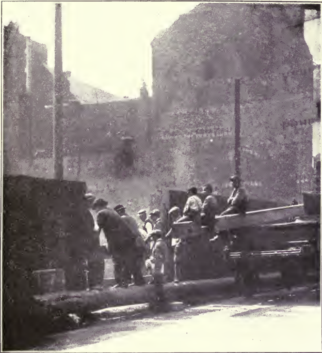
Boys who have left their youthful pursuits to watch the construction of a building
